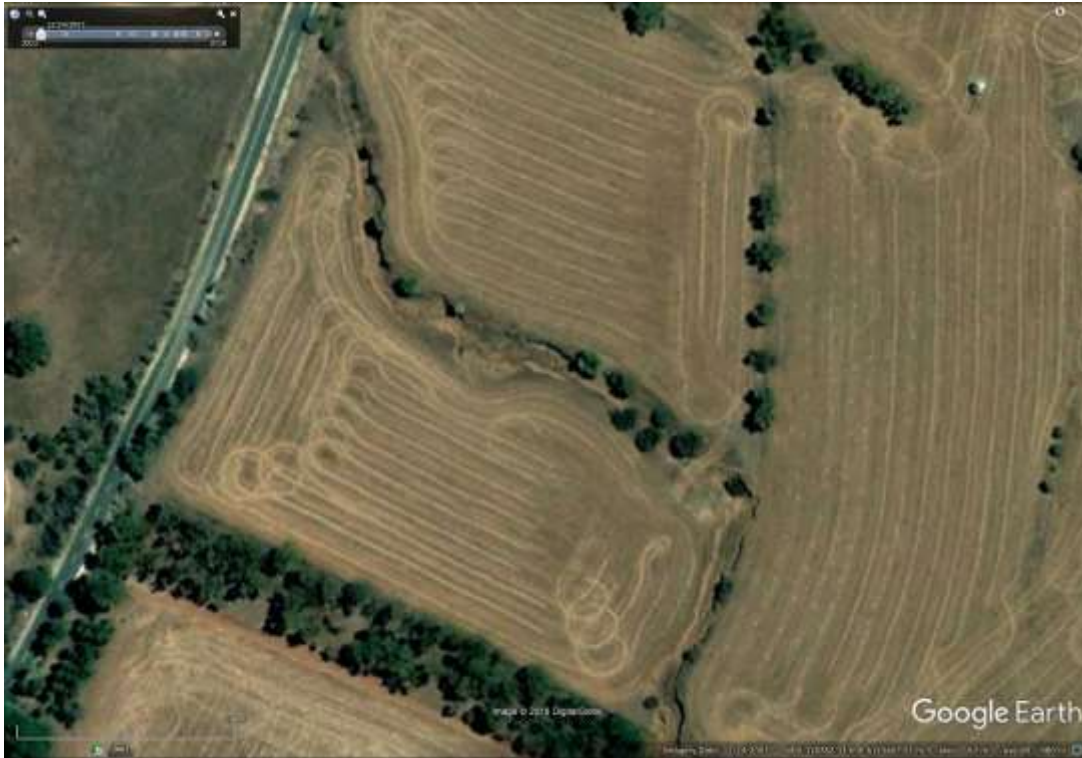
Figure 5E: December 2003 Google Earth image highlighting the erosion gully running through 141 Mine Rd. (mid-picture), “before rehabilitation”.
