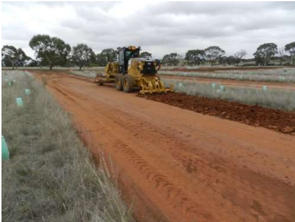
Figure 4: 141 Mine Rd; Deep-ripping subsoil following topsoil pre-stripping, between the rows which were pre-stripped and direct-seeded in 2015. Ripped areas (visible as the red-brown stripes in Figure 3 (above)), were cultivated and direct seeded with a diverse mixture of locally grown and collected native plant species in April/May 2018.
