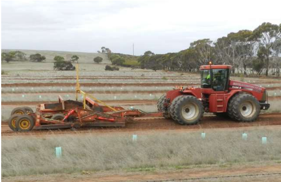
Figure 24: Picking up windrowed topsoil with a Case IH/ Land Plane combination – 141 Mine Rd.
