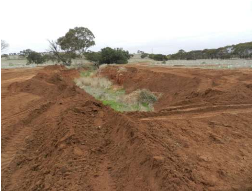
Figure 5C: East-West erosion gully during rehabilitation, 141 Mine Rd., May 2018
